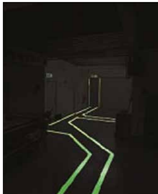
Figure 56: A way-guidance system
