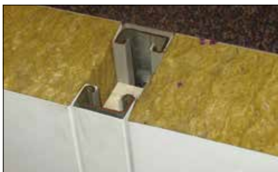
Figure 17: Insulated core panels - internal
