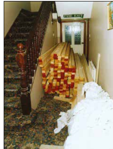
Figure 9: A blocked corridor with incorrect signage
